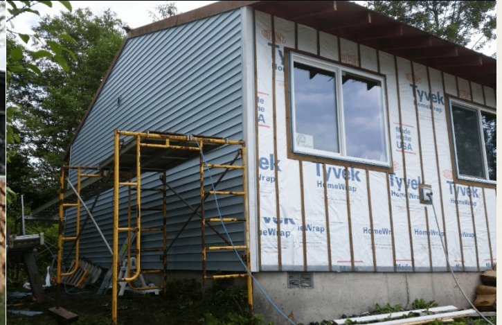
Siding replacement work in progress.
